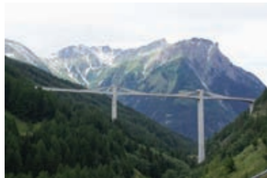
Figure 14. Ganter Bridge, Brig-Glis 1980
